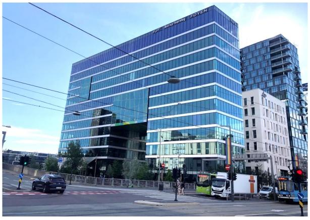
Figure 1: DEg 8, office building in Oslo, Norway, enveloped in quadruple glazed façade.
